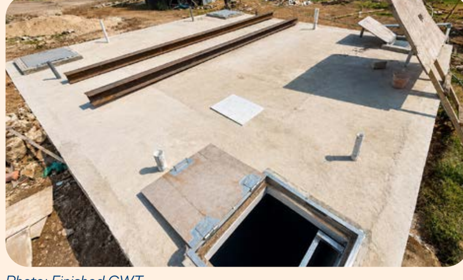
Photo: Finished GWT
